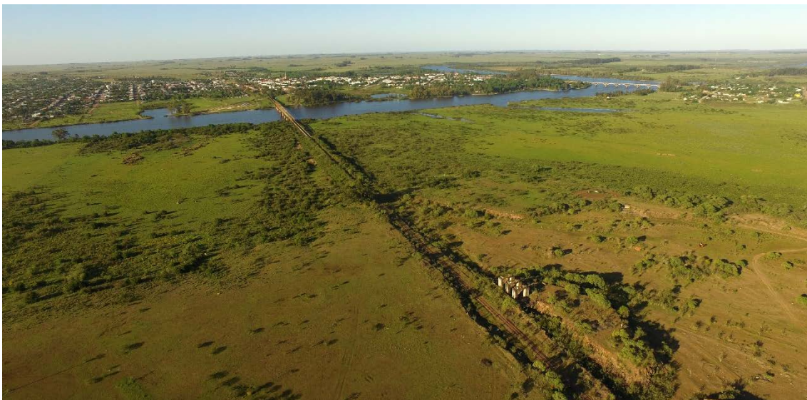
Quarry MTOP Q-008, discharge hoppers, railroad and Paso de los Toros city.
