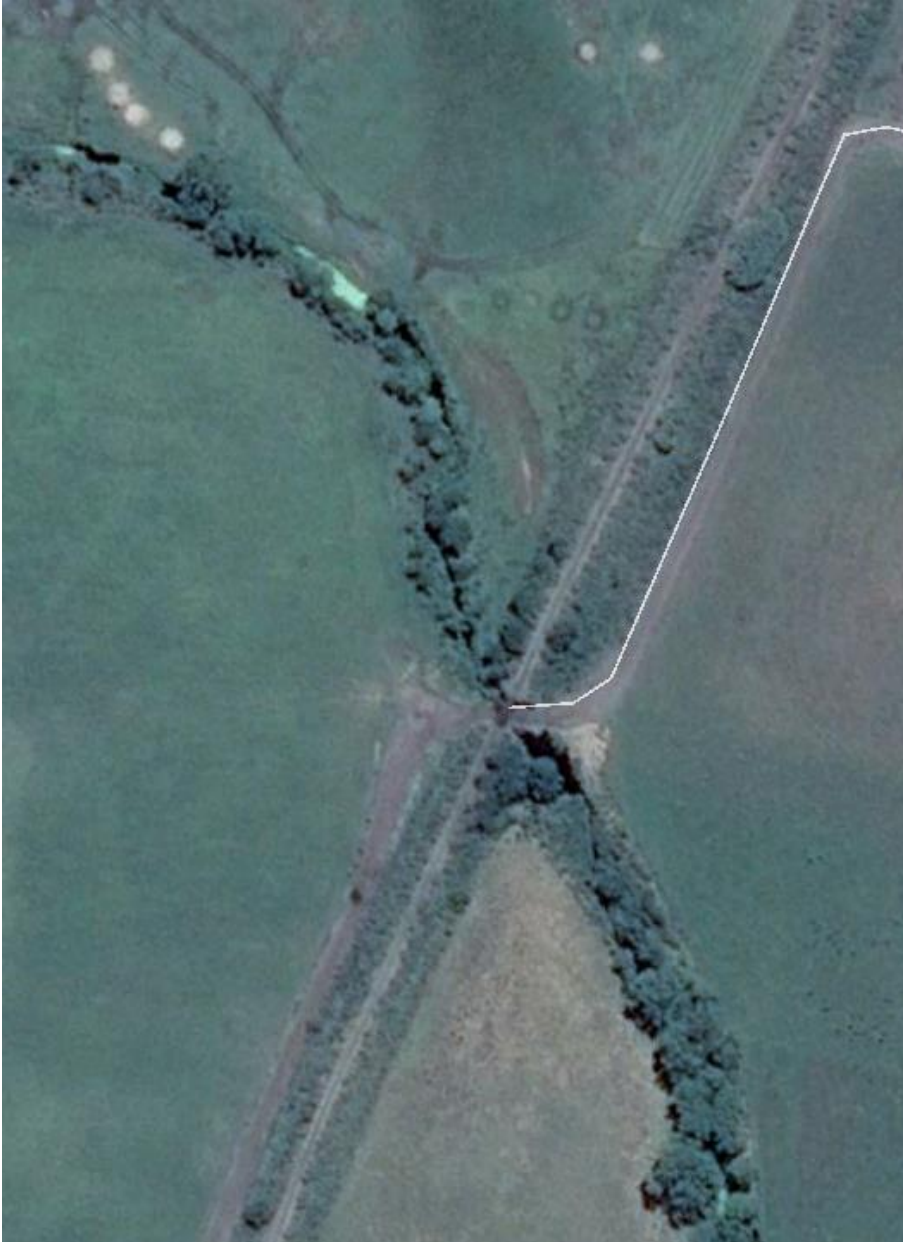
Figure 5-13 Railway embankment and stream vegetation
