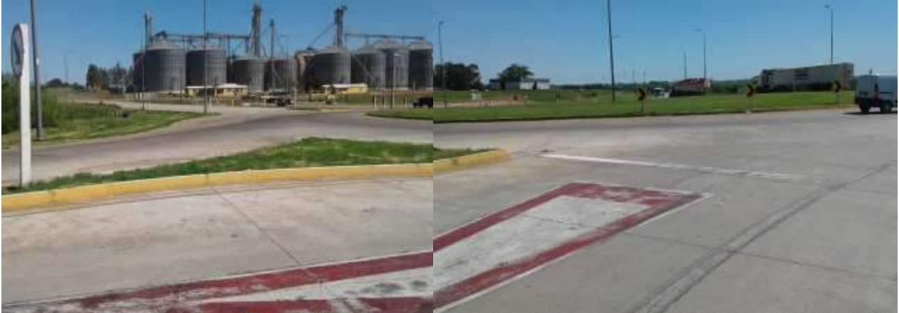
Foto 13.2-3 Vista By Pass Rotonda
